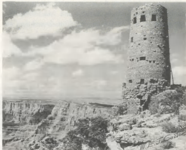
MARY E. J. COLTER, WATCHTOWER, ca. 1932, commercial photo signed by Mary E. J. Colter / WACHTTURM, signiertes Reklamefoto. (PHOTO: FRED HARVEY CO./GRAND CANYON NATIONAL PARK MUSEUM)
